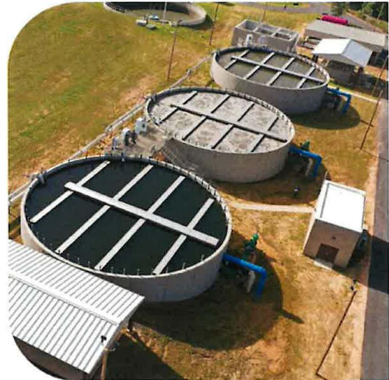
Aerial view of the AquaNereda® Aerobic Granular Sludge technology at the Wolf Creek WWTP in Foley, Alabama, in operation since January 2020
